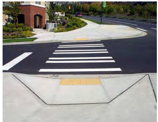
Curb Ramp NCDOT
