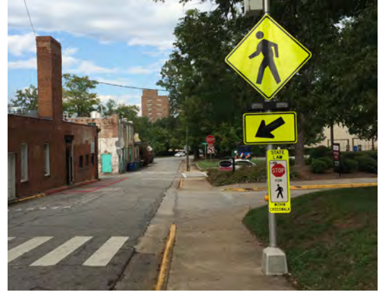
Pedestrian Signal - RRFB
