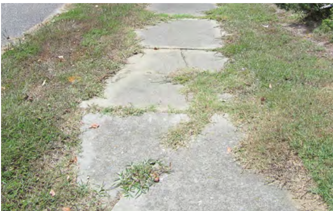
Inadequate sidewalks, such as those without curb cuts or those that are damaged, create accessibility challenges.
